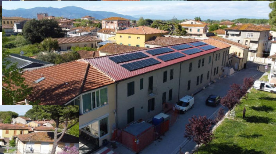
PONSACCO (PI) – 20 kWp
